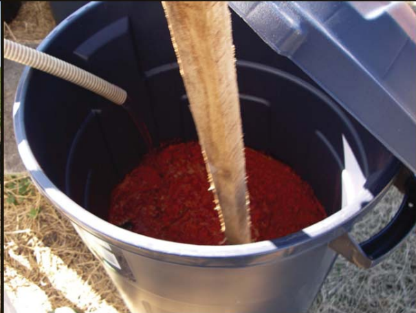
Mixing powdered AR92 into a container for injection.
